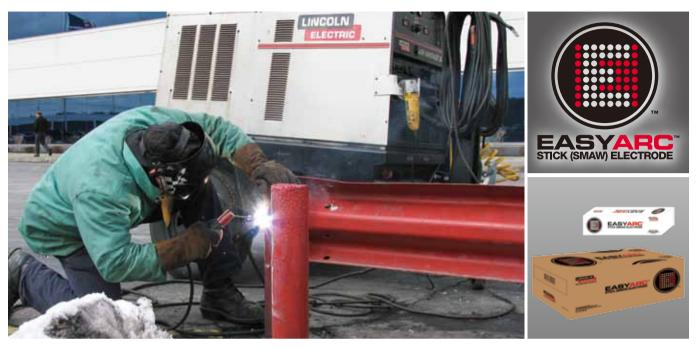
EASYARC™ 6013D is a rutile electrode, especially designed for vertical down welding of mild steel. It welds on AC or DC with excellent performance and easy restrike features.
